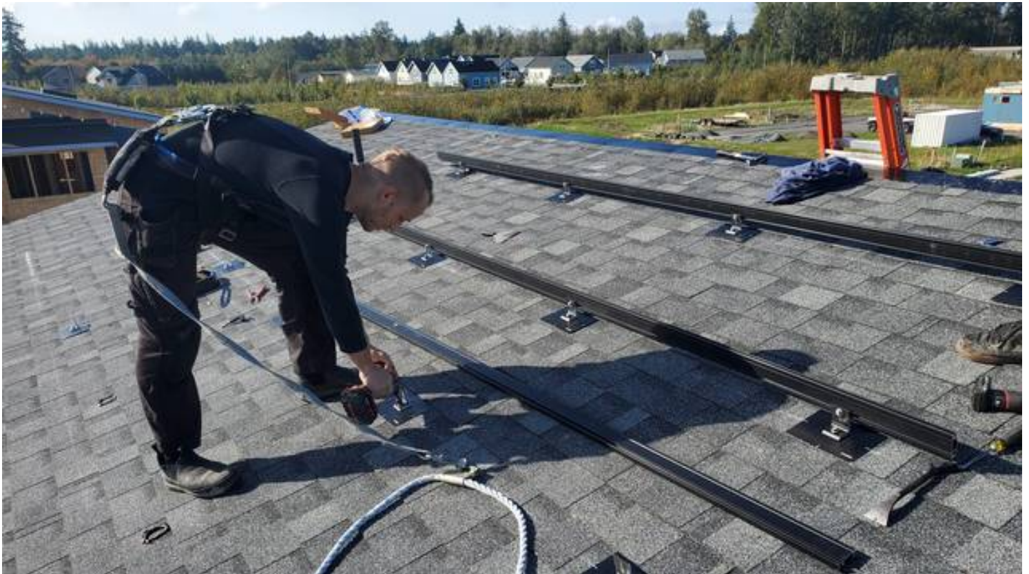
Corey Gittens of Velocity Electric installs frame mounts for solar panels on a new house in the Cordata area of Bellingham. Caitec, the developer in the area, has made solar panels a standard part of the new homes it is building in that area. STEVE DALRYMPLE, VELOCITY ELECTRIC COURTESY TO THE BELLINGHAM HERALD
